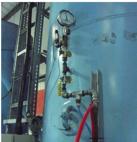
A “T-piece” at the air receiver pressure gauge port or in compressed air system piping are common sample points but do not provide accurate samples to test equipment and therefore must not be used.
